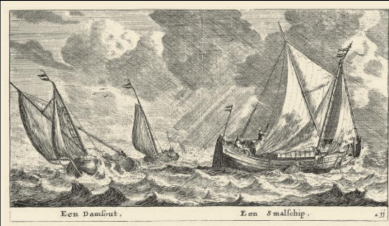
A Damsout and a Smalschip (the smaller sister ship of the *wijdschip*), etching by Reinier Nooms (1623-1664). A Damsout and a smallship looked alike and differed only in size. The *wijdschip* was also related to these types of vessel, which were used to load goods and to unload large ships. They could be taken on board.
